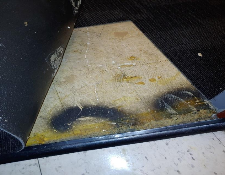
Two types of non-asbestos 12"x12" floor tile in Building 32/42.
